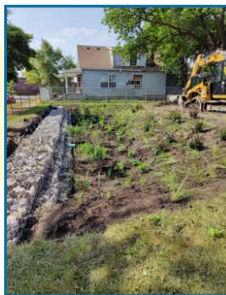
The rain garden in LaNita's pocket park prevents 116,000 gallons of rain water from flowing into Detroit's combined sewer system annually
