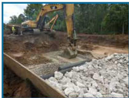
Fishway channel construction
